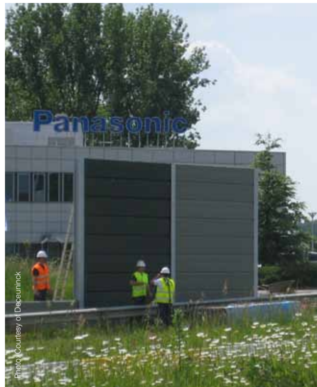
Sound barriers made of recycled PVC
