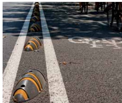
Traffic separators for cycle lanes made from post-consumer PVC waste
