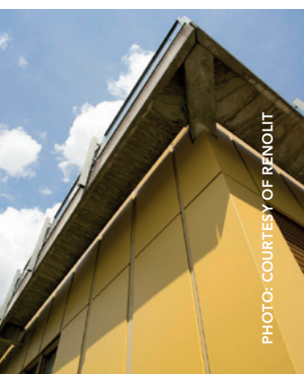
Anti-graffiti PVC films for facades facilitate buildings' maintenance.
