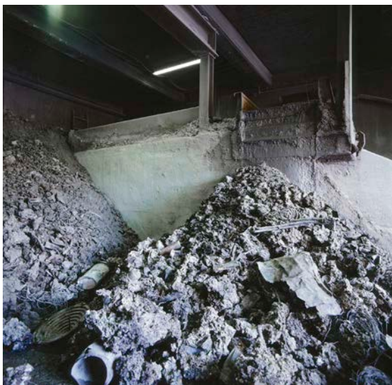
Incineration plant, Denmark
