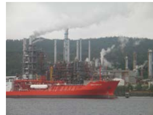
PVC plant, Norway
